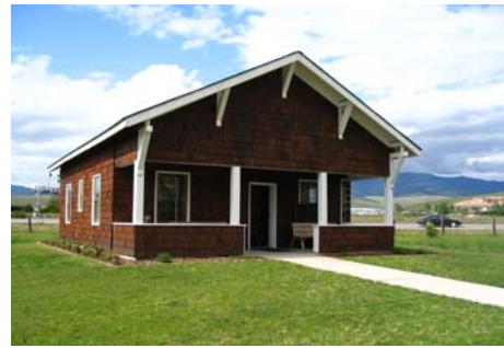
Bungalow Cabin Completed
